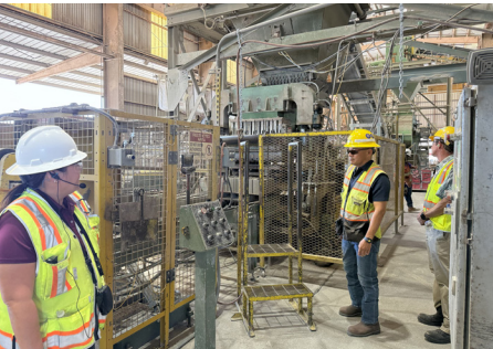
Vibration and compaction hydraulic
