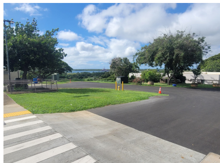
Leeward Community College, Flood Mitigation South End, Phase II
