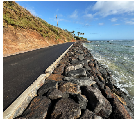
'Aliomanu Road Repairs by Oceanit
