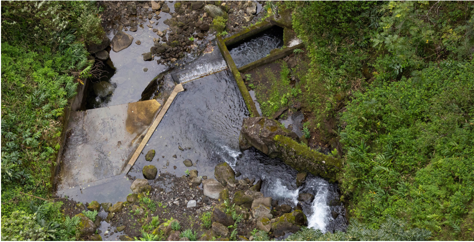
Lower Hamakua Ditch - Waipio Valley Miscellaneous Improvements by Engineering Partners, Inc.
