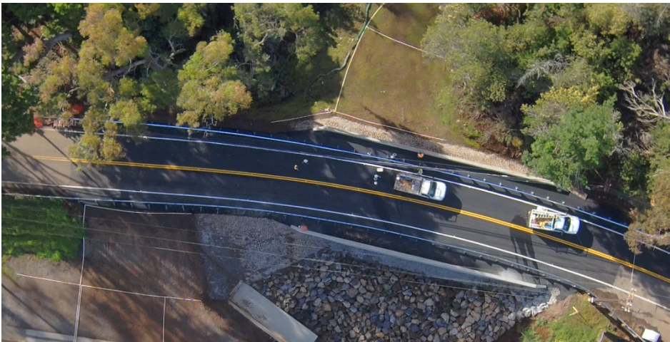
Kekaulike Avenue, Emergency Repairs M.P. 8.2
