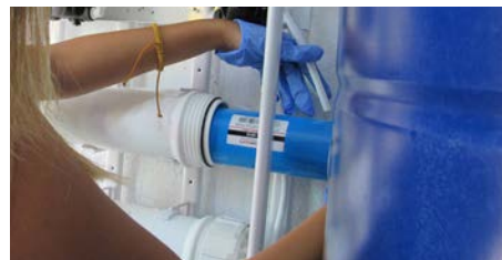
Installing the filters
